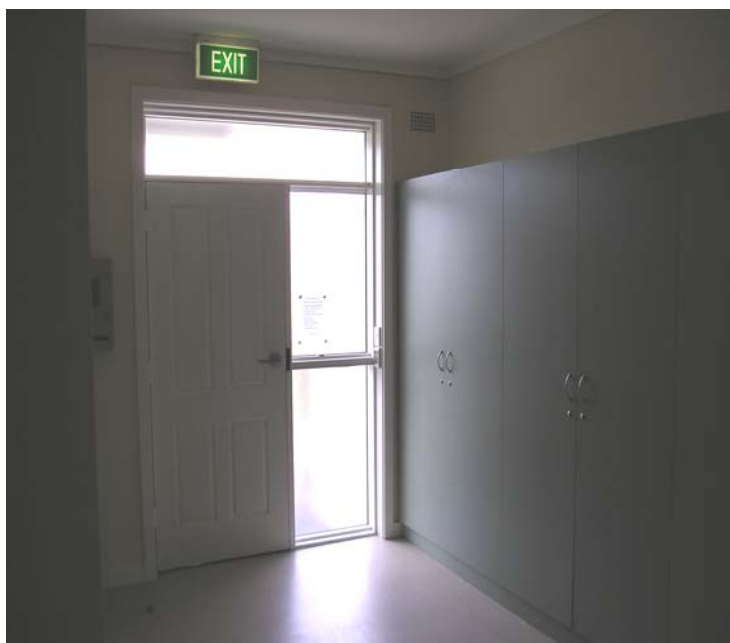
Figure 14: The sidelights allow in natural light and the cupboards provide additional lockable storage
