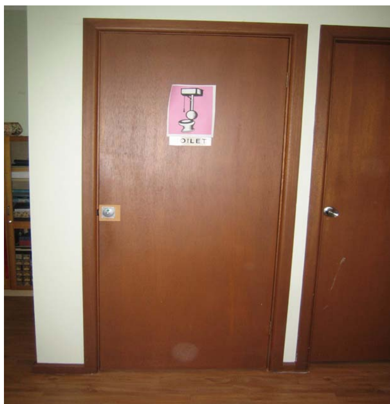
Figure 9: The toilet door has a large picture and large occupied indicator.
